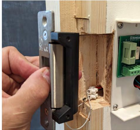
**17. Refit the electric strike and carefully feed the cables through the door frame.**
