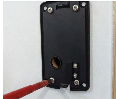
**12. In this instance we will use the rubber gasket.** Place the gasket over the pre-drilled holes and then align the backplate over the gasket. Fix to the wall using the 4 included fixing screws.
