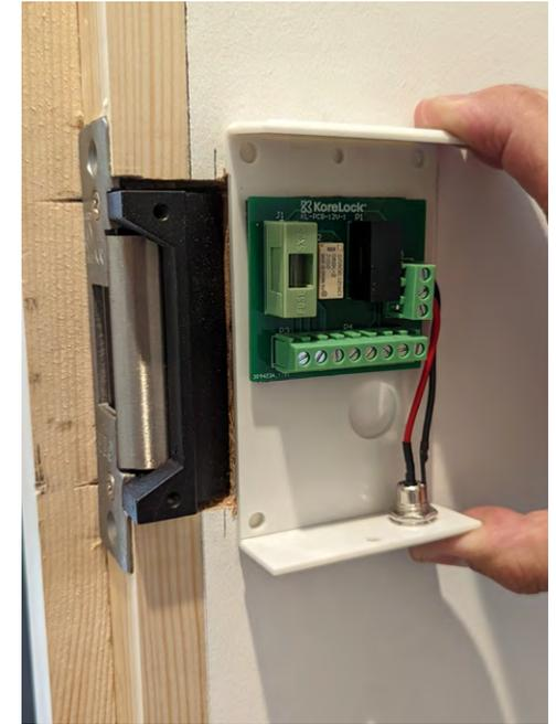
**4. Position the white enclosure in the preferred position.** In this instance we will install it close to the strike. This wall is hollow so the keypad and enclosure do not need to align exactly on the internal and external walls. If the wall is solid then it might be easier to drill a hole through the wall so they align perfectly. You will need to make sure that the cables from the electric strike have a route to the enclosure.
