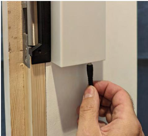
**23. Plug the 12V adapter into the jack on the underside of the enclosure and then plug the adapter into the main power supply.**
