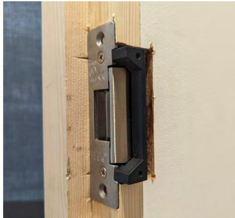
**2. Prepare electric strike install.** Determine the best position for the electric strike. Prepare the frame with the proper size cutout to fit the strike as per manufacturer's instructions.
