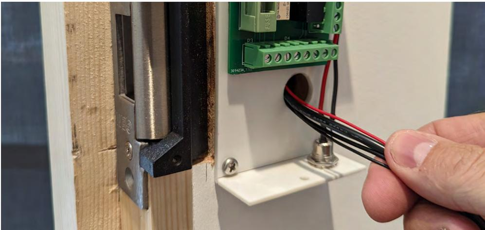
**18. Locate and carefully pull the cables through the hole in the white enclosure.**
