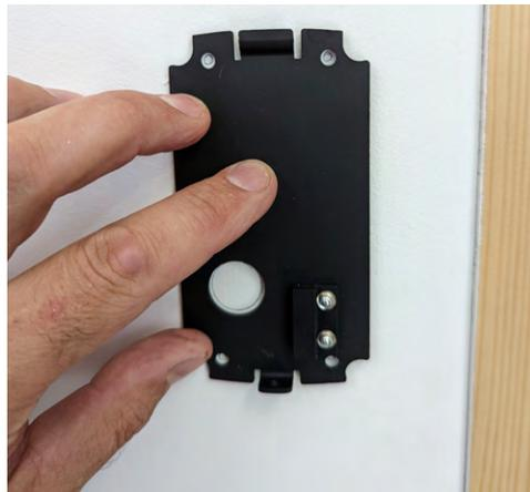
**8. Position the keypad backplate and mark the position of the cable and fixing holes.**
