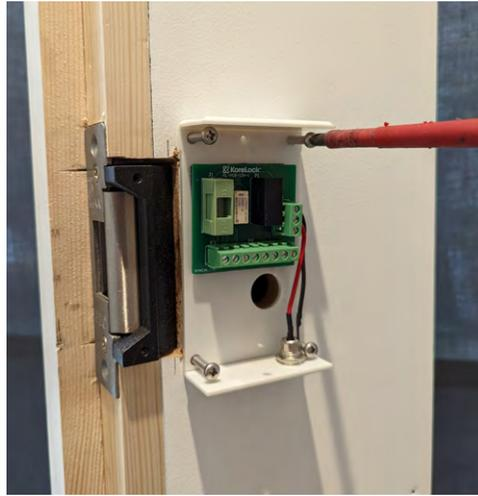
**6. Fix the enclosure to the wall using the included fixings.**
