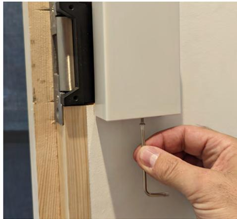
**22. Snap the enclosure cover back on, making sure that no cables are pinched.** Secure in place using the T10 security screw and wrench.
