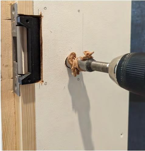
**5. Mark the position of the cable and mounting screws and drill a 3/4" (19mm) cable hole.**
